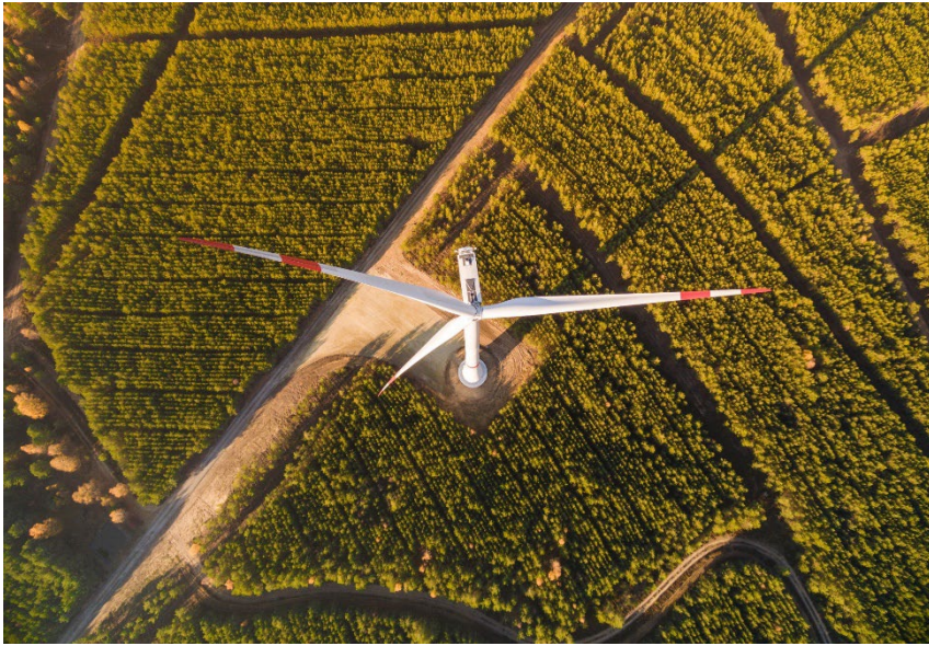
© FA Wind/Janto Trappe; Windpark Chransdorf, Brandenburg
